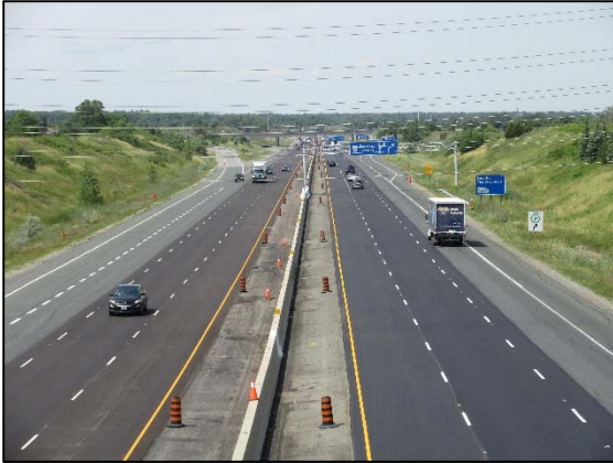
July 2019. Looking east with CUM1-1a communities north and south of 407ETR.
