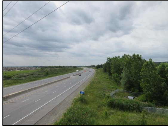
July 2019. Looking southwest at CUM1-1a and a hedgerow within the 407ETR right-of-way, just west of Walkers Line.
